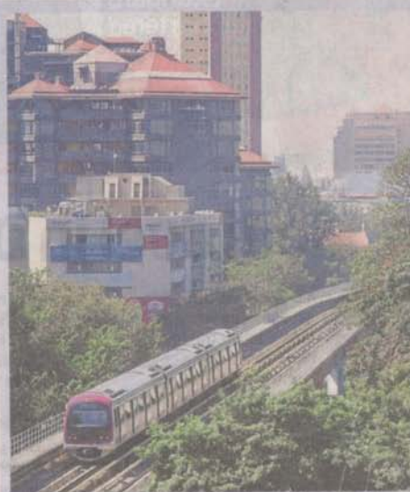
The BMRCCL has sought central funding for the ORR metro line (Phase 2A) and the airport line (Phase 2B). DH FILE PHOTO
